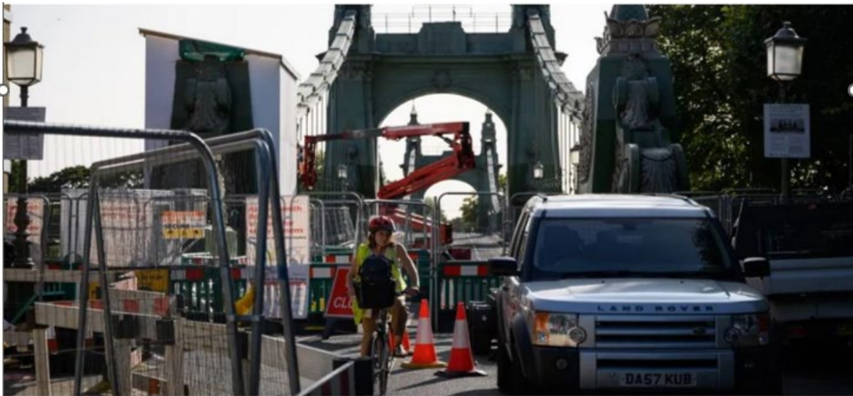
Figure 1: Hammersmith Bridge under repair since 2019
